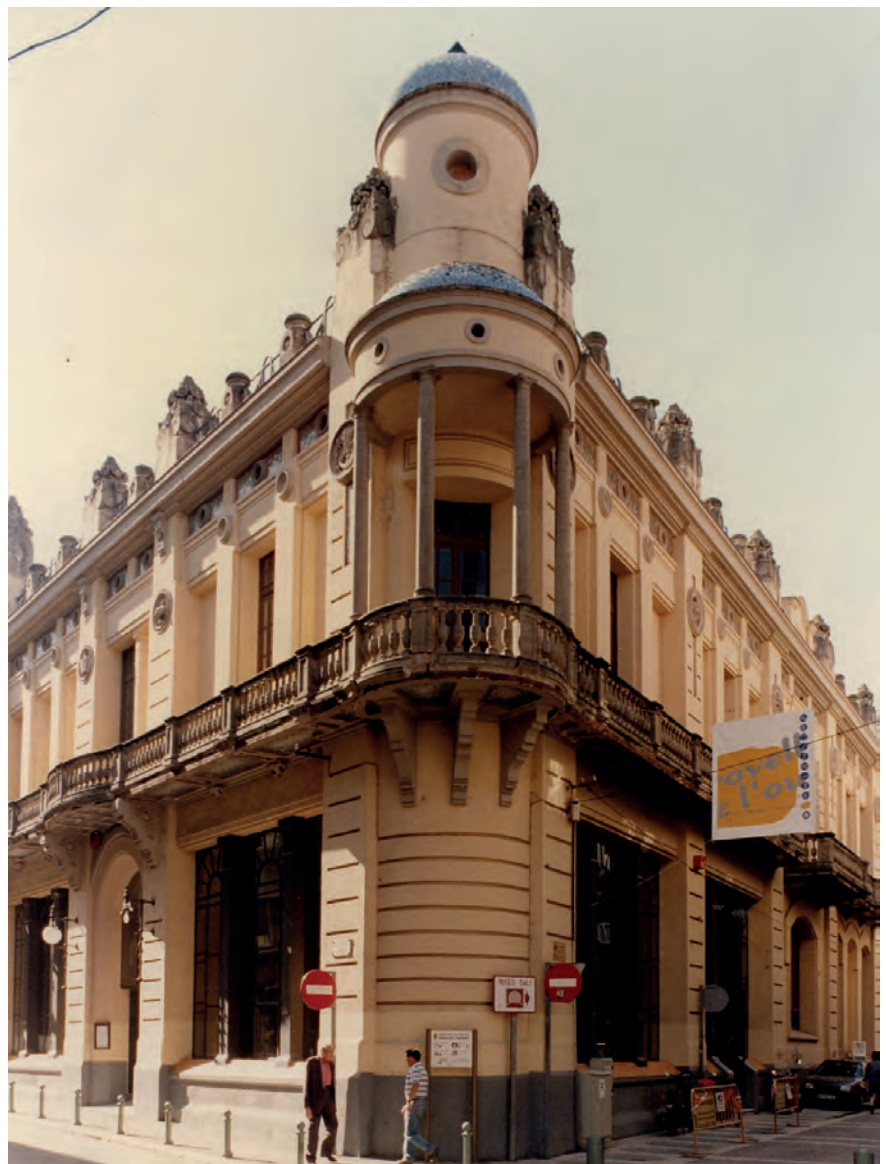
FIGURE 2. Building that houses the headquarters of the Casino Menestral Figuerenc (Tradesmen's Recreational Society of Figueres), designed by the architect Josep Bori i Gensana (1904). It is listed in the Inventory of Architectural Heritage of Catalonia.
